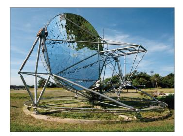
• CSP parabolic dish systems use mirrors that are mounted over a parabolic-shaped dish to focus the sun's rays onto a receiver. The receiver is positioned at the focal point on a nearby structure along with a heat engine, which has thin tubes inside it. The tubes contain a gas, such as helium or hydrogen, or even air. The system, which can attain very high temperatures, is equipped with a tracking system that follows the arc of the sun.
